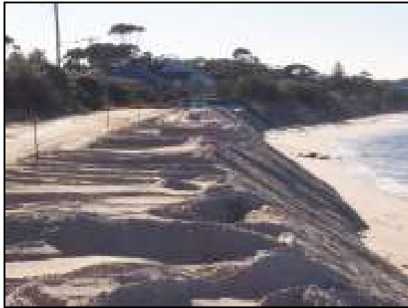
Figure 6a: Emergency dumping of sand to save the road at Jimmys Beach during June long weekend (Courtesy Department Environment & Climate Change)
